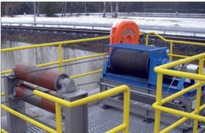
SB-E 304 as a traversing winch for a water treatment plant
