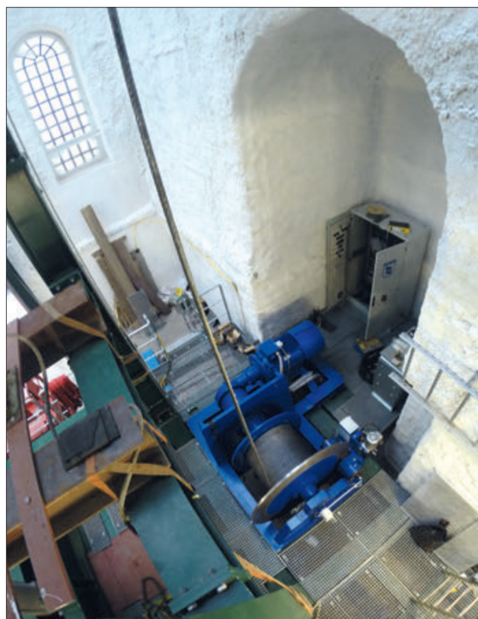
SB-E 316 as a hoist winch for a pump line
