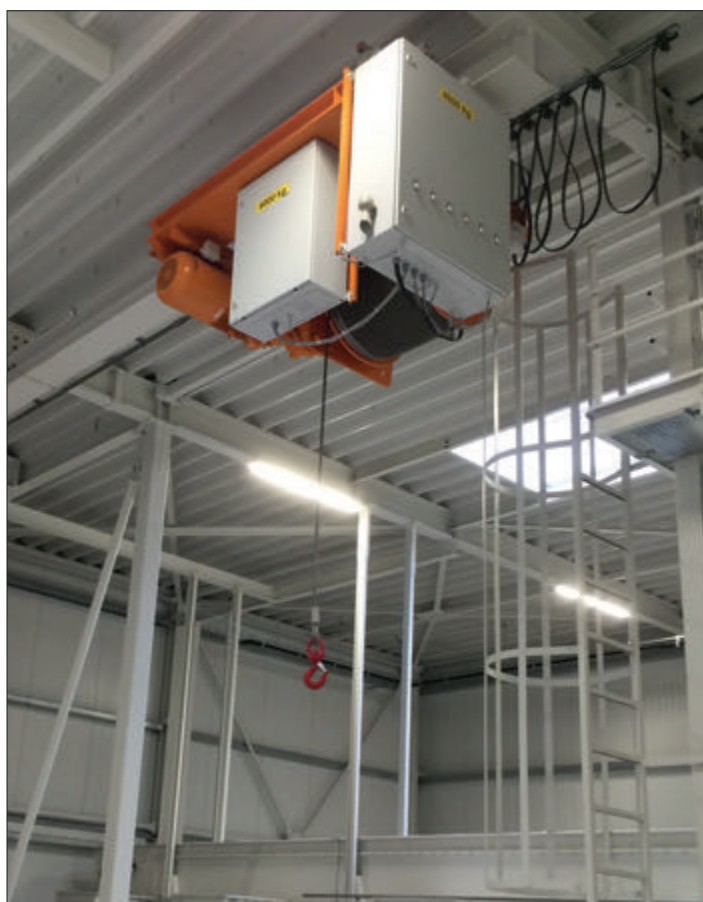
SB-E307 as a mobile rope hoist
